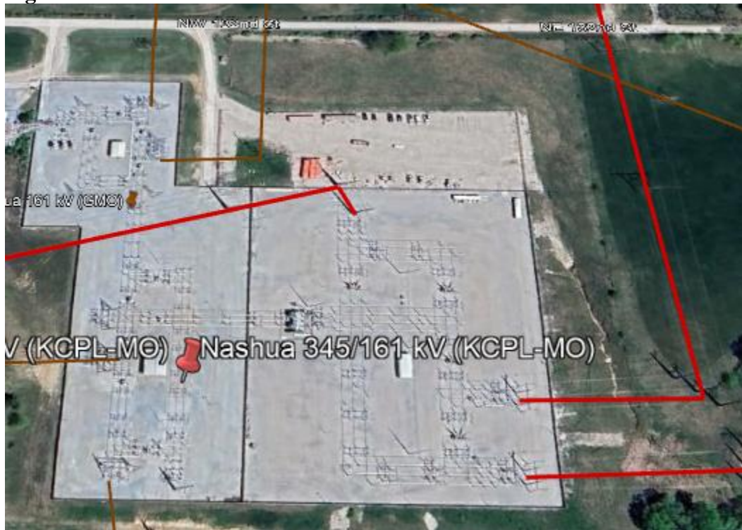
Figure 2 – Nashua 345kV Sub
